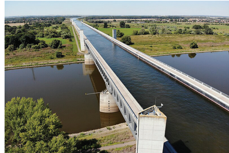
Magdeburg Water Bridge, Germany. Source: Wikimedia Commons, Olivier Cleynen.
