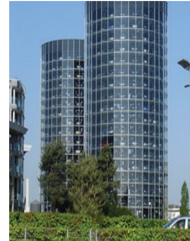
Storage Silo, Wolfsburg, Germany. Source: Flickr, Saskane.
