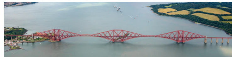
The Forth Bridge (Cantilever Bridge), Edinburgh, UK. Source: Wikimedia Commons, MrMasterKeyboard.
