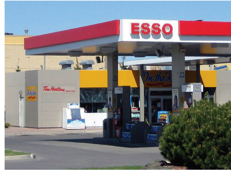
Esso Gas Station - On The Run store brand. Source: Wikimedia Commons, Stickguy.
