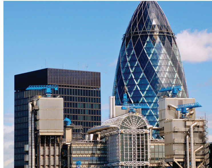
The Gherkin and the Lloyd's Building, London. Source: Openverse, It's No Game.
