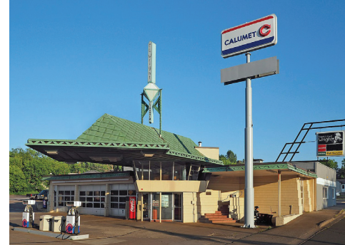
Lindholm Oil Company Service Station, Cloquet, USA. Source: Wikimedia Commons, McGhiever.
