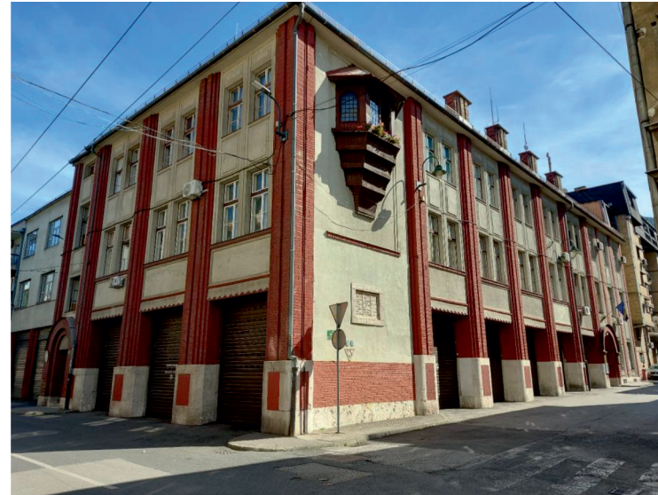
Fire station in Sarajevo, BiH. Source: Authors
