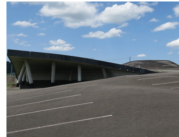
Hybrid parking, Tokamachi, Niigata, Japan. Source: Wikipedia, Qurren.
