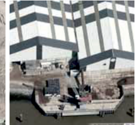
Quay - crane - storage
