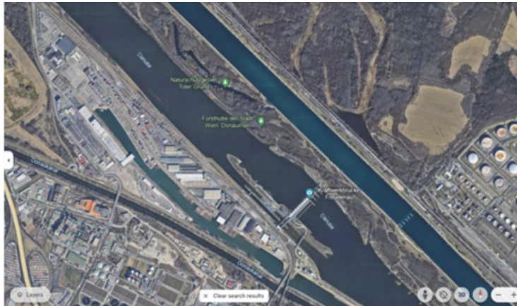
Port of Vienna, Austria. Source: Google Earth.
