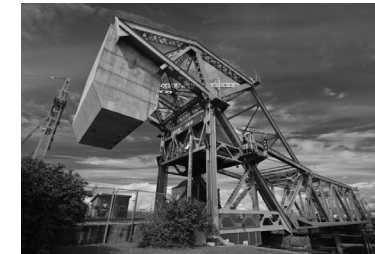
Skansen bridge, Trondheim, Norway. Source: Flickr, Superlangbein.
