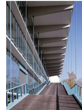
Car parking, Düsseldorf, Germany. Source: Baukunst.
