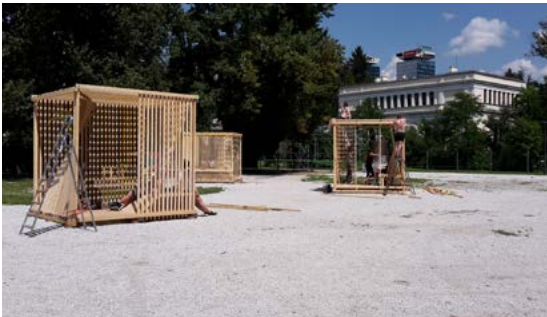
Picture 8 – Work in progress (Authors)
