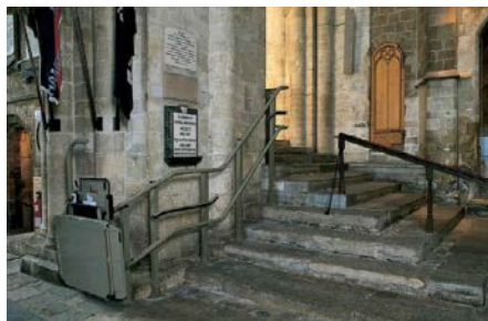
Sl. 499 - Stepenišna platforma instalirana u Winchester Chatedral, Hampshire, Engleska
