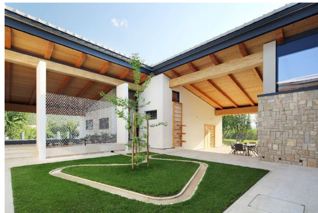
Figure 4: House VLHS, central atrium with the tree and the element of water © Anida Krečo.
