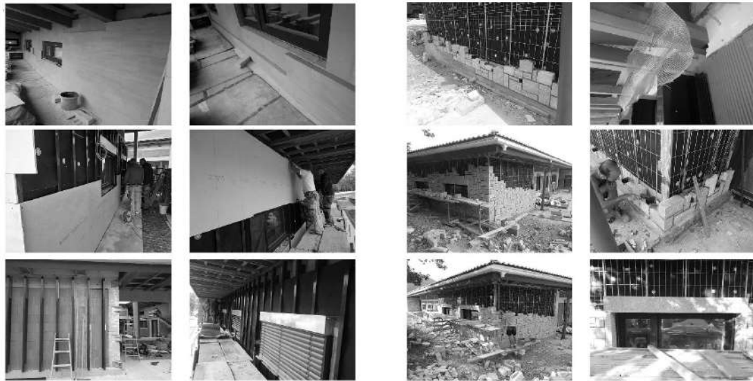
Figure 8: House VLHS, construction phase details © Vedad Islambegović.
