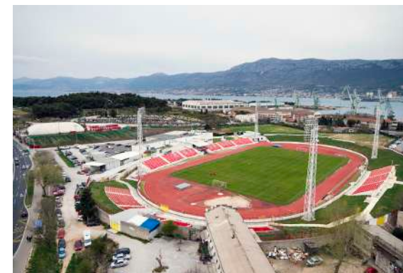
Figure 9: Aerial view of the Stadium “RNK Split” in the Youth Park (source: RNK Split webpage. Last accessed June 17, 2021. https://rnksplit.hr/klub/stadion ).
