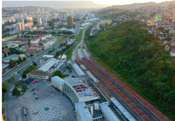
Figure 18. Top: Railway station. Centre: Radio and television headquarters. Bottom: Old electrical power plant.
