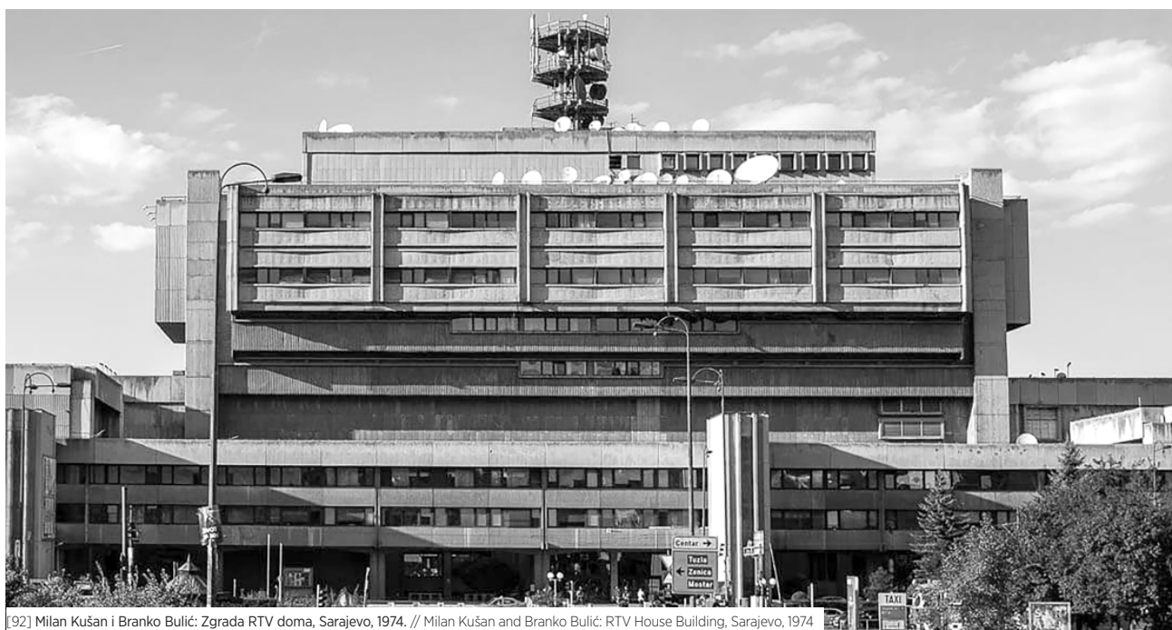
[92] Milan Kušan i Branko Bulić: Zgrada RTV doma, Sarajevo, 1974. // Milan Kušan and Branko Bulić: RTV House Building, Sarajevo, 1974
