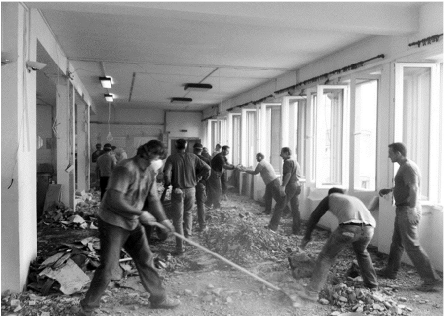
Figure 34-Demolition phase © Vedad Islambegovic
