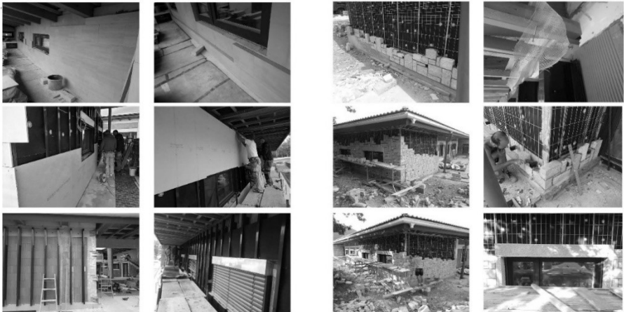
Figure 66- construction process © Vedad Islambegović
