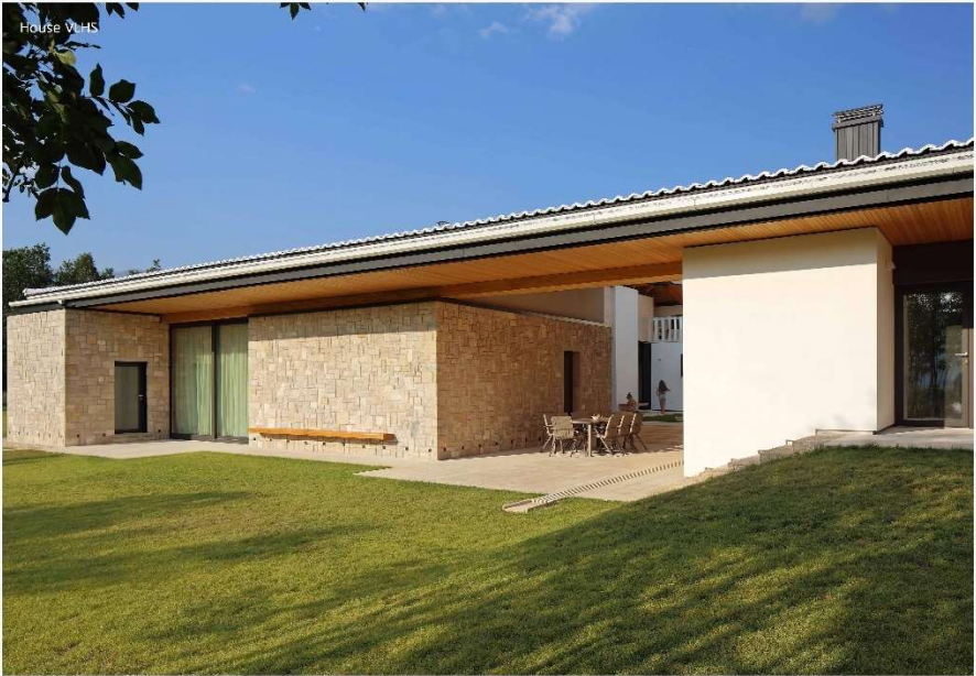
Figure 62- south-west elevation with the roof eave © Anida Kreco
