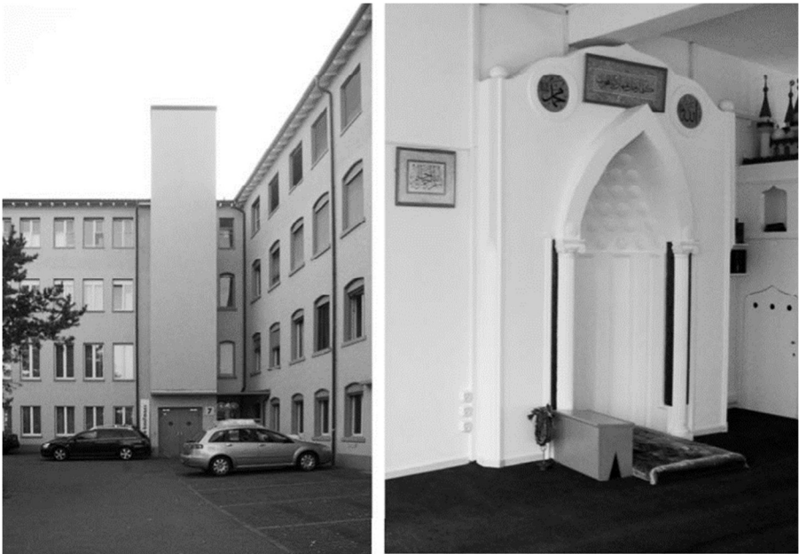
Figure 24-existing industrial building and the Prayer Hall before renovation © Vedad Islambegovic
