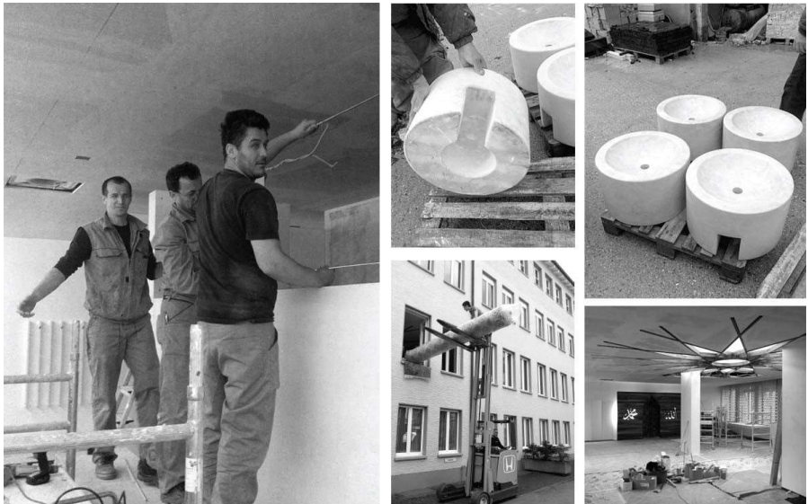
Figure 35- Different phases of construction © Vedad Islambegovic
