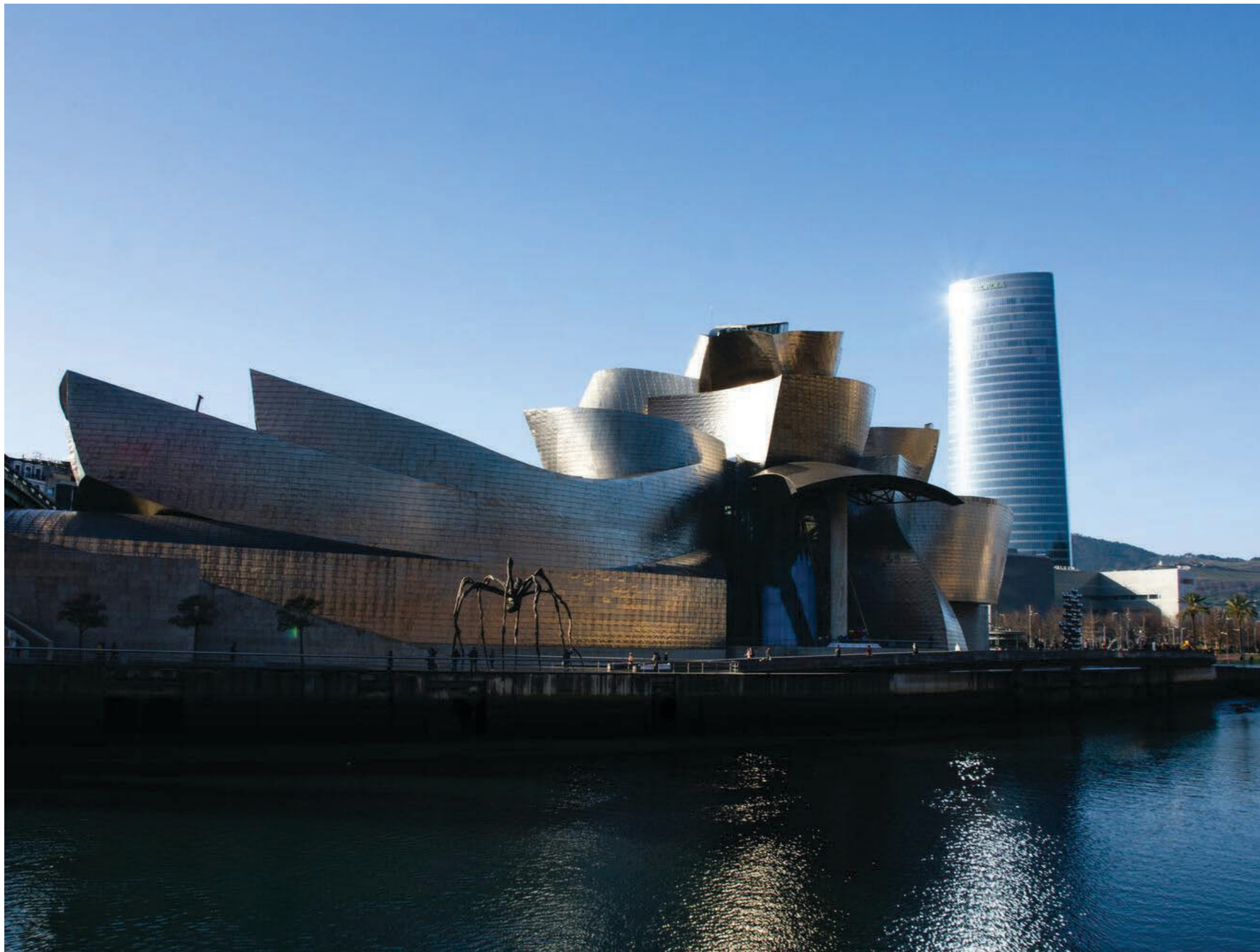
Image 64 Exterior appearance of the Guggenheim Museum Bilbao
