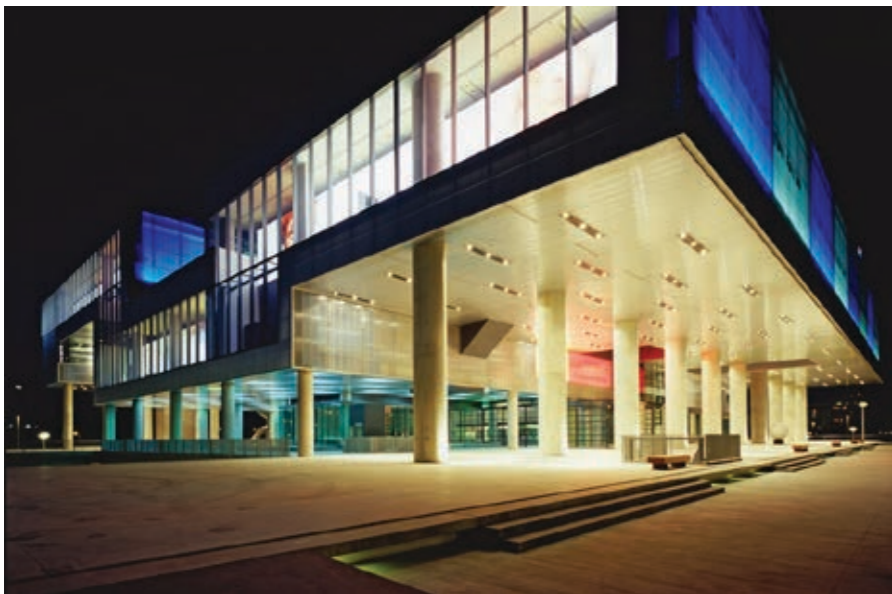
Image 103 Exterior of MSU Zagreb, west façade
