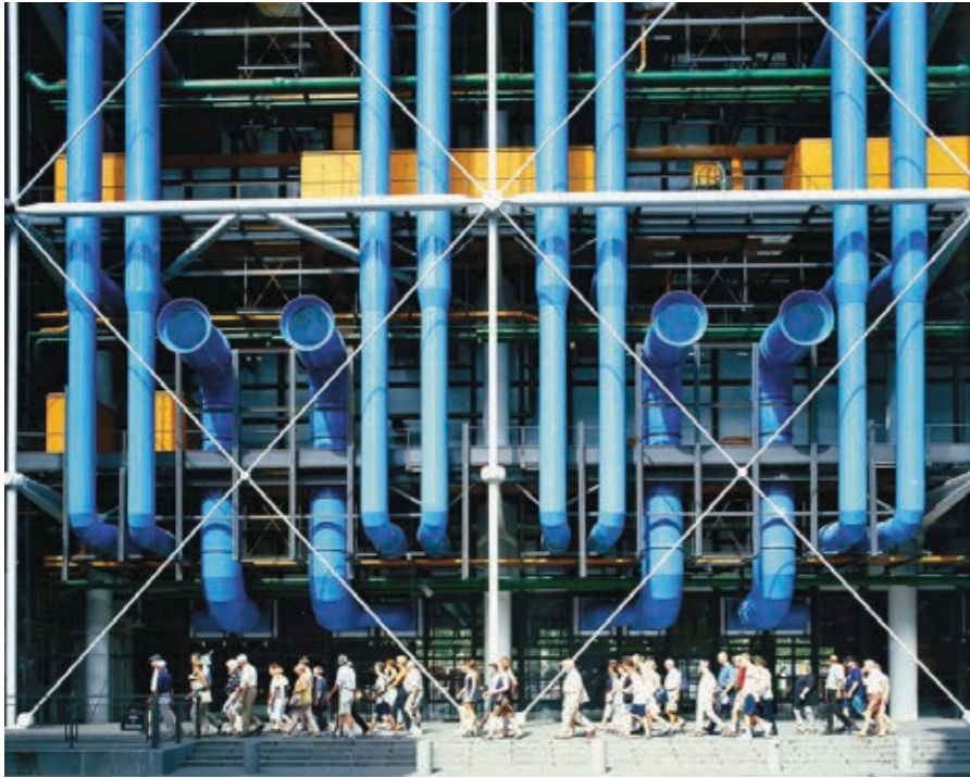
Image 83 View of the facade detail (installations)
