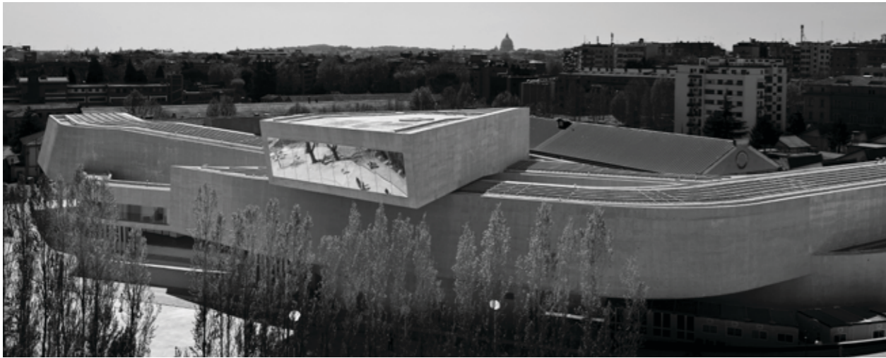
Image 66 Exterior appearance of the MAXXI museum complex
